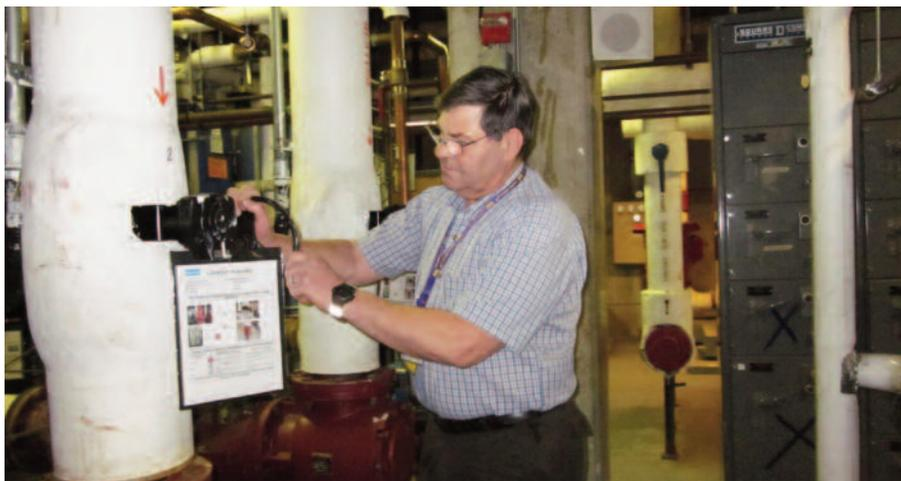
Jack Grexton, engineer, Building Services, in the main boiler area, closes off the Apotex heat circulating valve to carry out preventative maintenance to the pump. With the implementation of our new computerized management maintenance system, Facilities Services engineers will be notified when preventive maintenance work such as this needs to be done.
